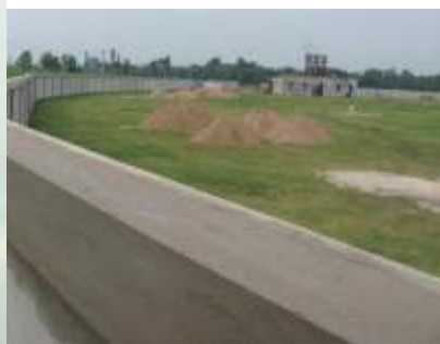
Completed compound wall
