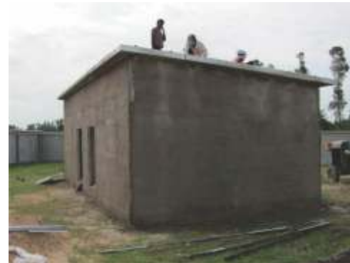
Above: Sunrise Orphanage's new office building taking shape
